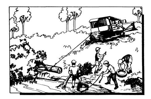
4 Key Standard No. 21: Construct water bars on skid tracks and decommissioned roads Construct water bars on skid tracks near log landings and watercourses.
